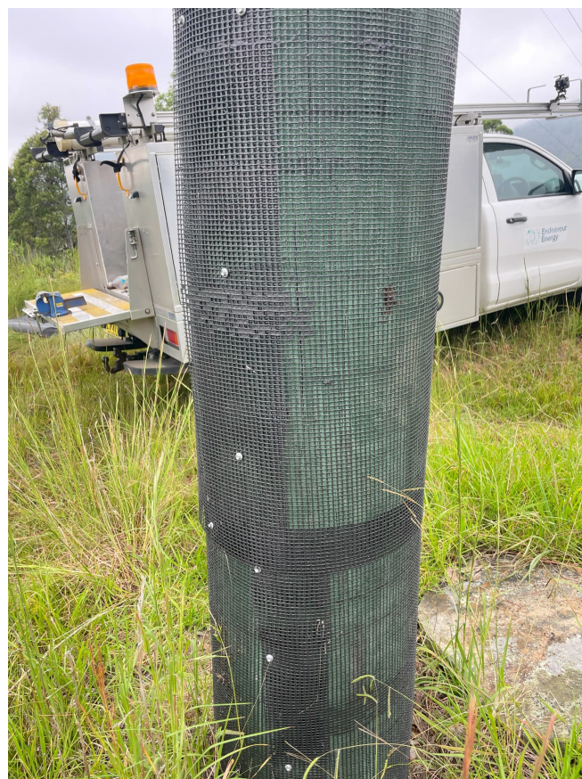
Figure 2 - Fire Mesh wrap installed on CCA pole.
