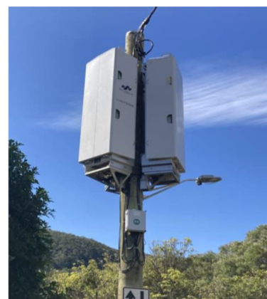
Photo: EcoJoule 'EcoStore' 85kWh 40kVA output (Gen 2)
