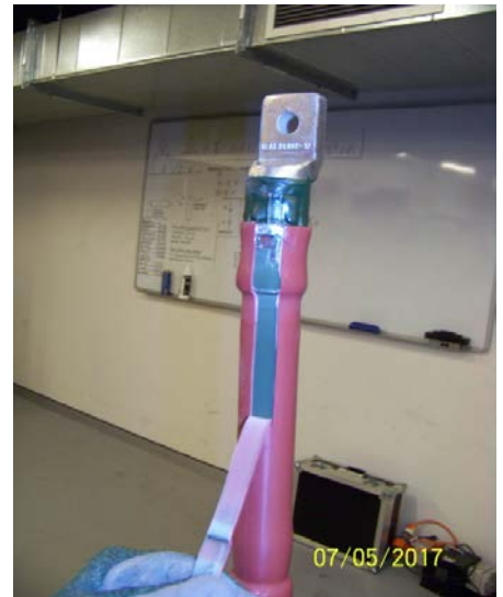
Figure 7: Soft blue flame. Pre-heat lug barrel and post heat lug palm and the entire termination length until the length starts to contract, a bead of mastic appears around the lug barrel at the top of the insulation tube and a thin band around the bottom edge of the tube. Note the green mastic has bonded to the XLPE and lug so well it could not be peeled away
