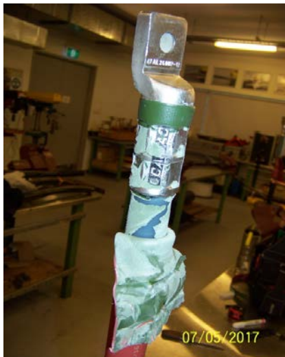
Figure 6: Pre-heat lug barrel and post heat lug palm. Soft blue flame for 4 mins until a thin bead appeared top and bottom of the insulation tube
