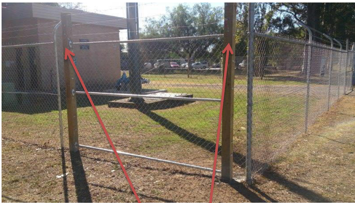
Correct customer isolation but no danger signs installed
