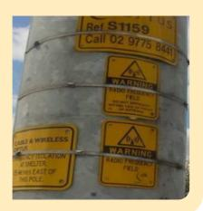
Radio emissions pose a potential danger. Care must be taken to avoid approach to these installations until isolated in accordance with approved procedures.
