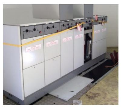
Figure 14 – "Barrier "out" method for the erection of a barrier on totally enclosed switchgear
