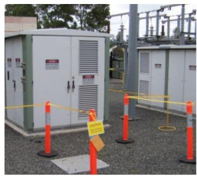
Figure 13 – Barrier "in" method for the erection of a barrier in a substation
