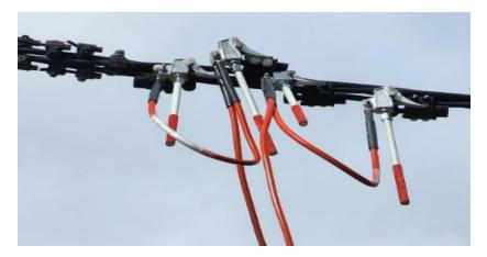
Figure 26 – Example application to overhead ABC mains
