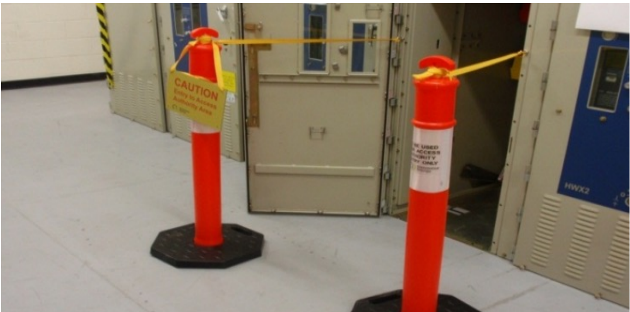
Figure 11 – Example of switchgear under Access Authority with yellow tape defining entry area
