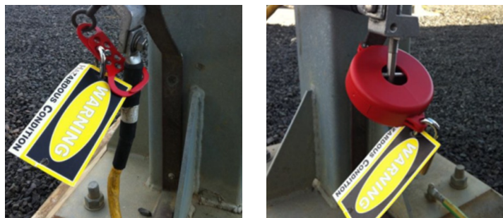
Figure 15 – Example locking mechanisms
