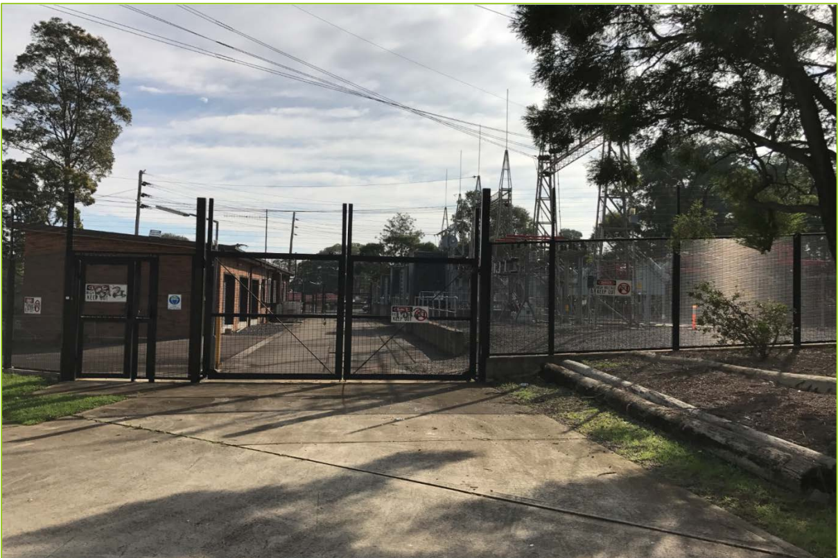
Figure 6: A northerly view of the Marayong ZS from Frederick Street.
