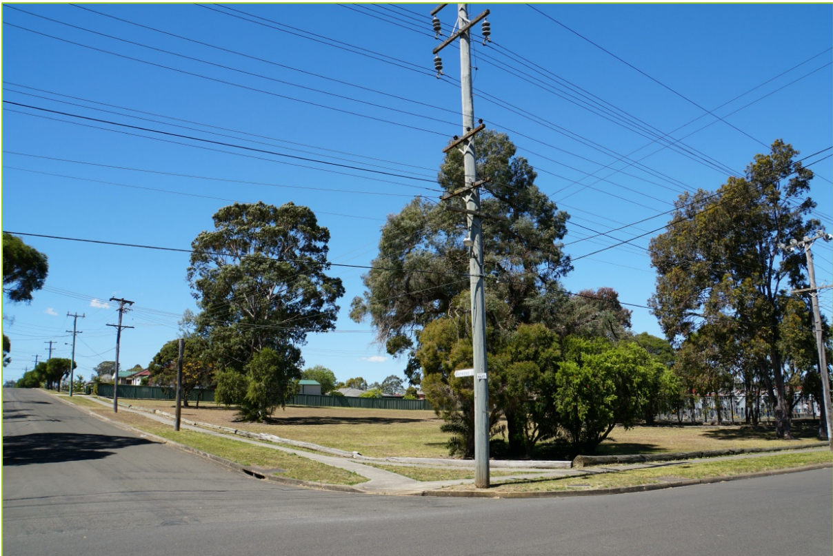
Figure 4: A southeast view of the subject ZS site from the corner of Raymond and Charles Street (photo by design consultant).
