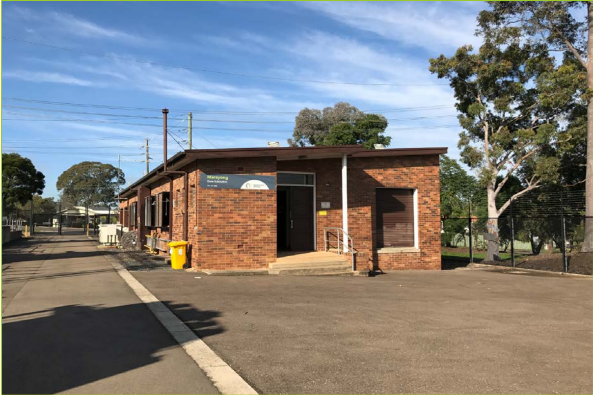
Figure 7: A southerly view of the existing Marayong ZS Control Building that is to be demolished.
