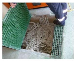
Figure 11: Cable pit subject to flooding
