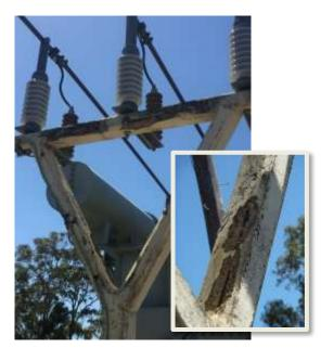
Figure 10: Corrosion damage on the ZS's support structures
