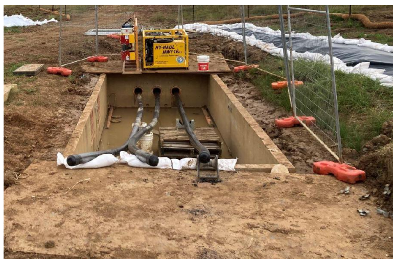
Figure 7.4 Typical joint bay during construction
