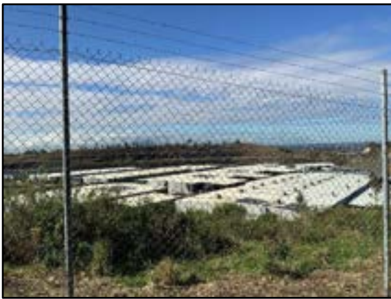
Figure 21. View from the proposed location of the new works, facing south-east
