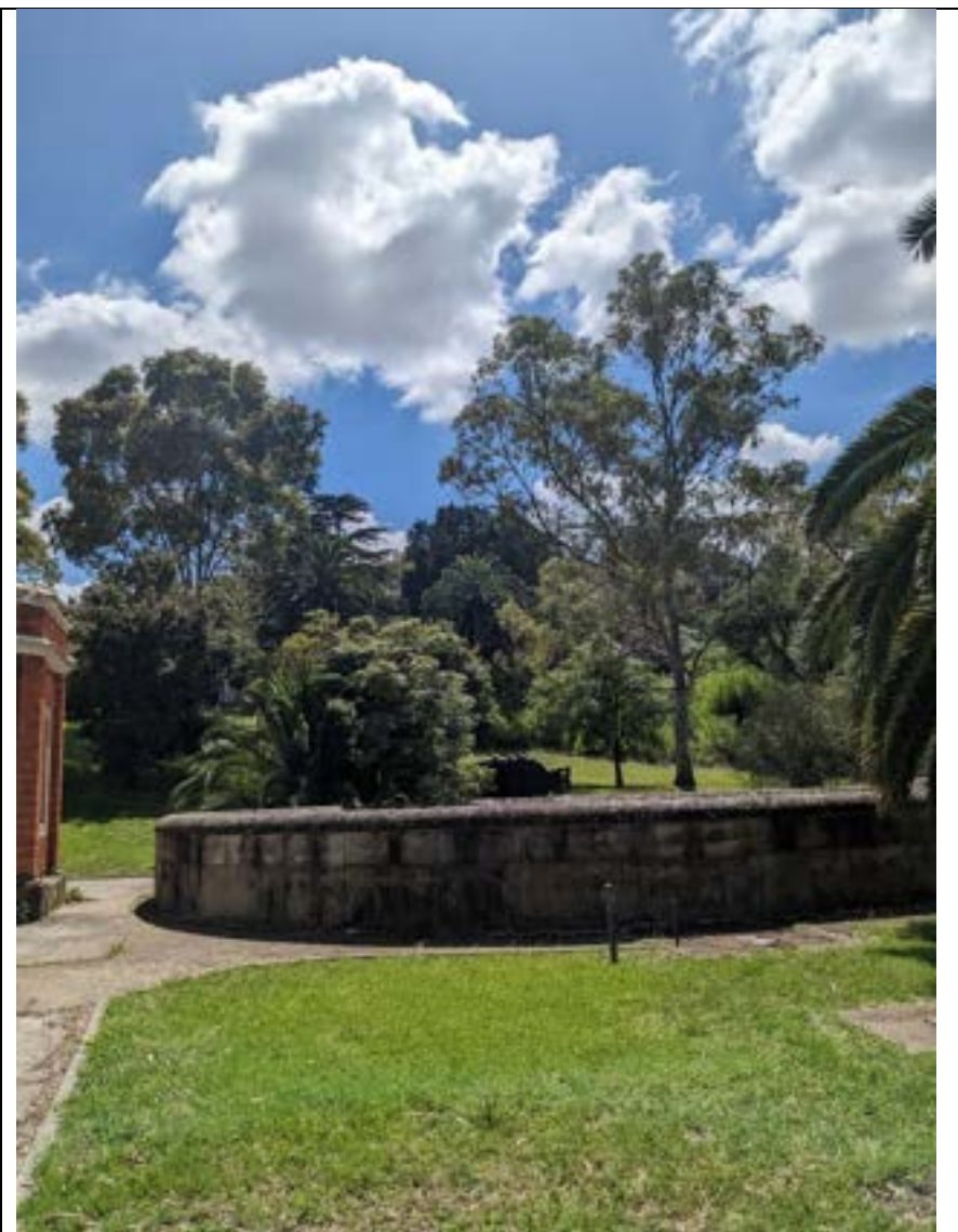
Figure 4. View towards tower location from Valve House
