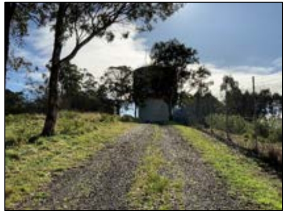
Figure 16. View from the proposed location of the new works, facing north-east towards two elevated reservoirs
