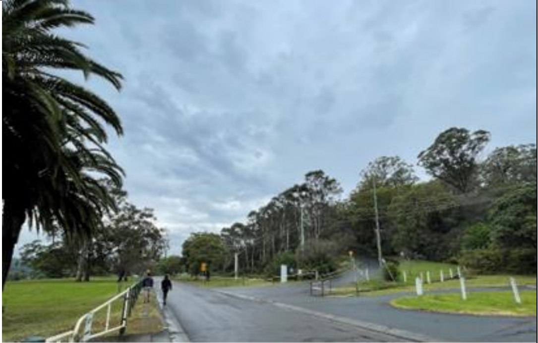
Photo I – View from gateway adjacent submerged tower and in close proximity to Prospect Reservoir Valve House, looking up road to picnic areas and George Maunder Lookout on Prospect Hill.
