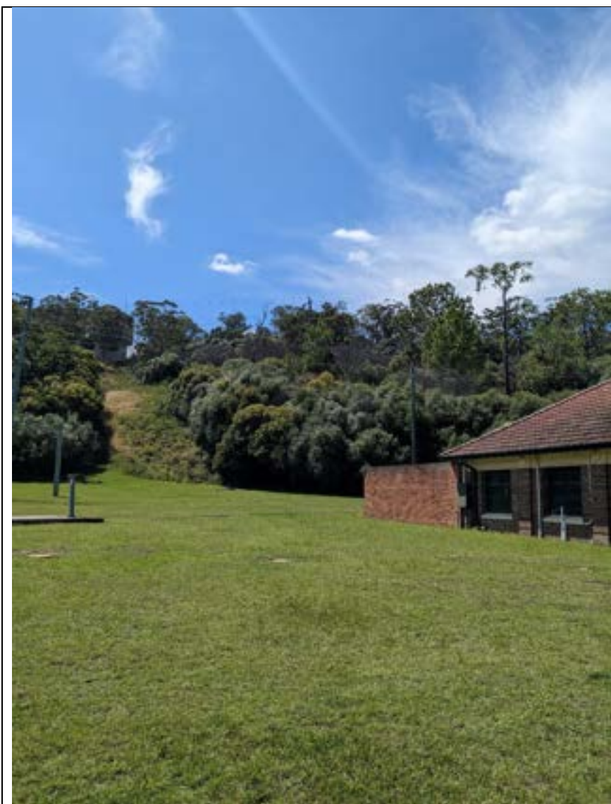
Figure 3. View of tower location from vicinity of Sydney Water offices
