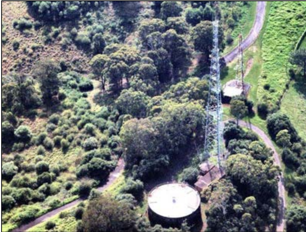
Figure 26. Aerial imagery of an existing tower (Waterboard Tower at Horsley Park) which is similar in design to the proposal. (Source: Image provided by Endeavour Energy, 9 November 2022)
