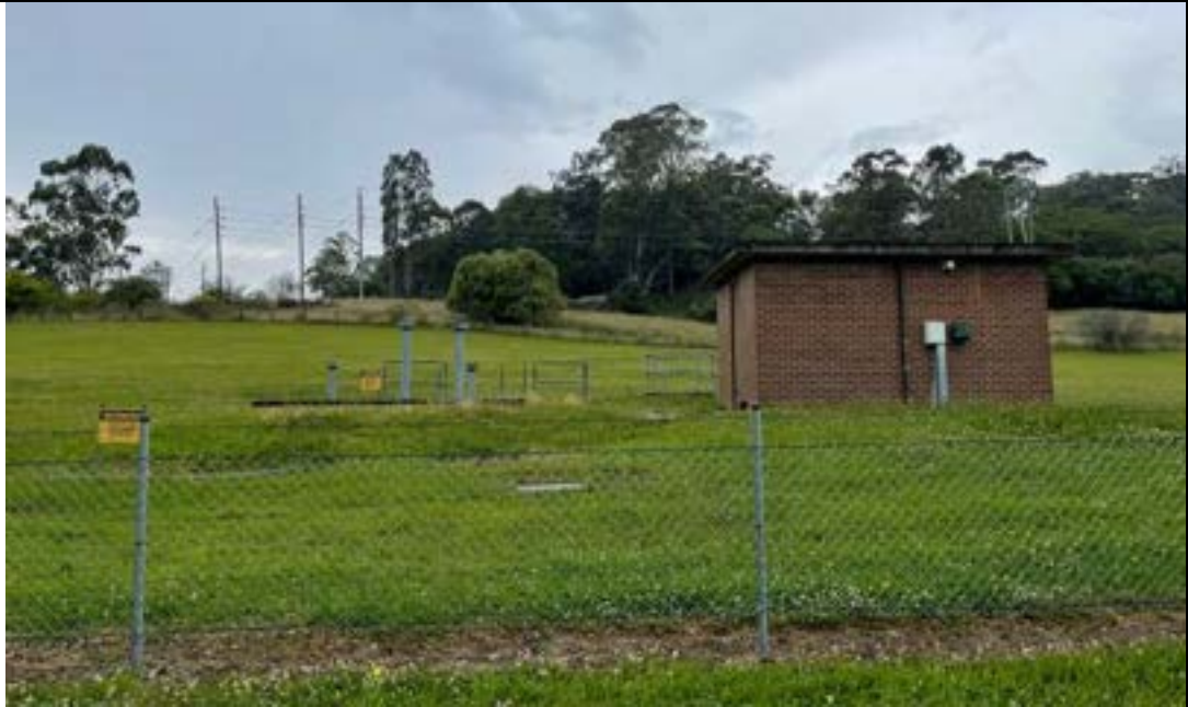
Photo F – view towards existing power lines from William Lawson Drive.
