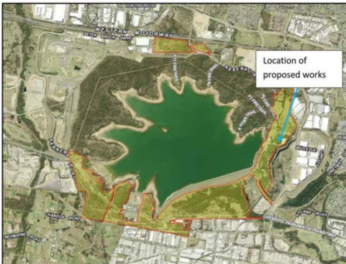
Figure 1: Aerial view of the Prospect reservoir site highlighted in yellow (source: sixmaps).
