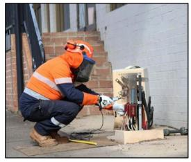
Routine external inspection of LV terminations in LV pillars and streetlight columns include external thermal inspection using infra-red camera (conducted every 4 years).
