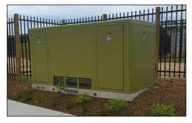
Endeavour Energy assets are predominately located in the public domain, including approximately 14,500 padmount substations, of which more than 98% are fibreglass cubicles.
