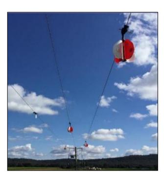
This advice may also incorporate the implementation of critical controls such as isolations, aerial markers and installation of temporary insulation (also known as tiger tails or tarapoli) to enable third party workers to safely build and operate on scaffold and, where required, use cranes to lift over the network.
