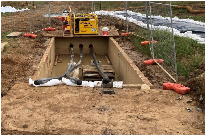
Figure 7-12 Joint bay during construction
