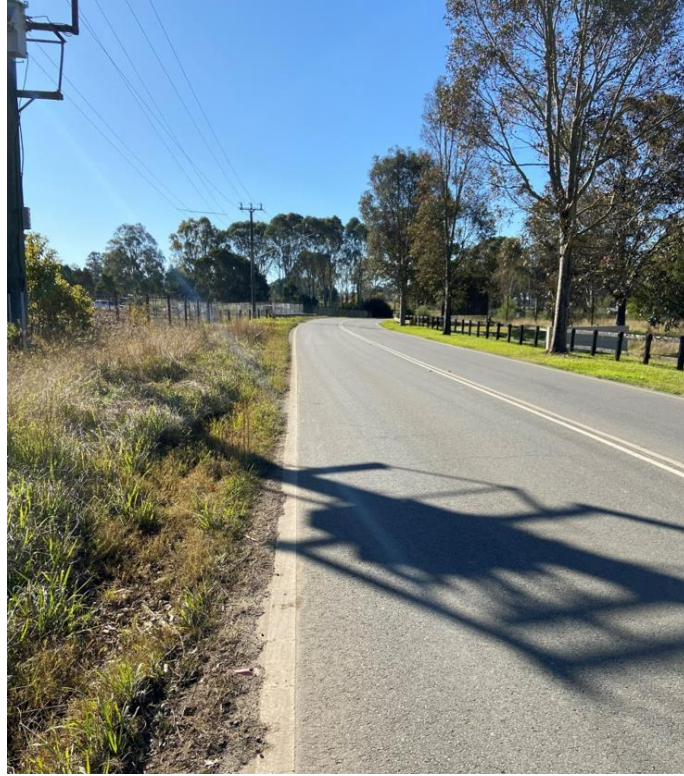
Photograph 6.1 North facing on Luddenham Road at joint bay JB 28
