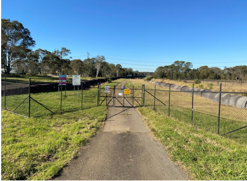
Photograph 6.3 East facing from Luddenham Road along Warragamba pipeline
